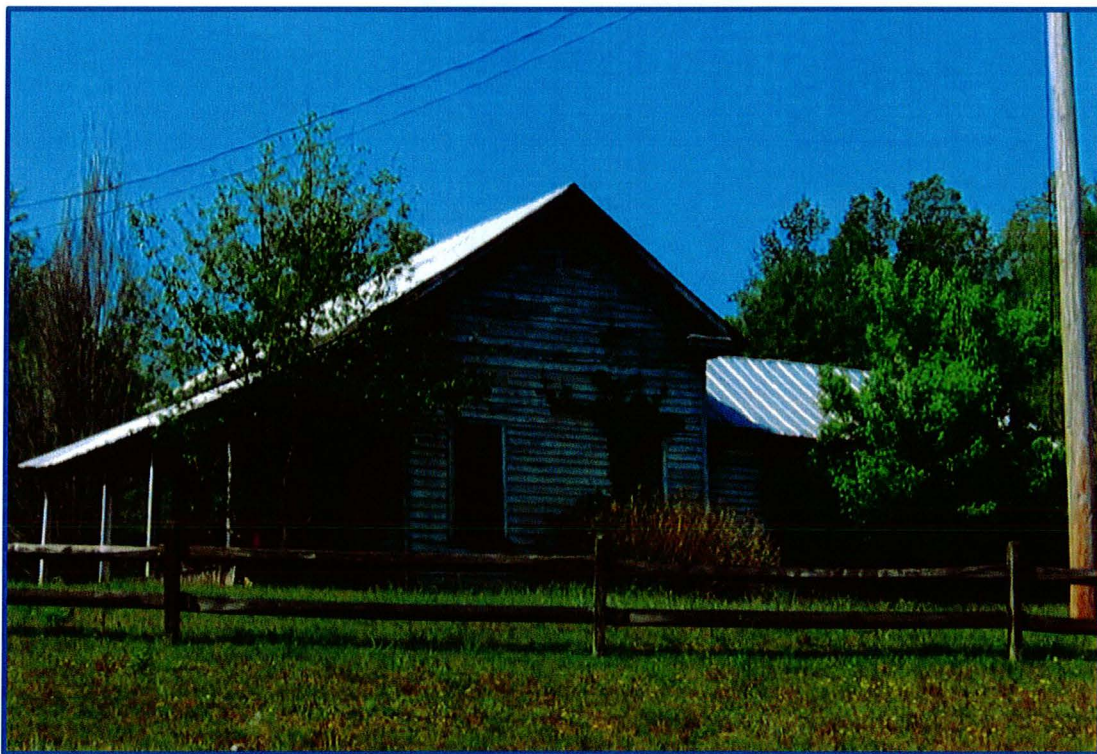
Figure 6. Dwelling house. East (main) and north elevations.
