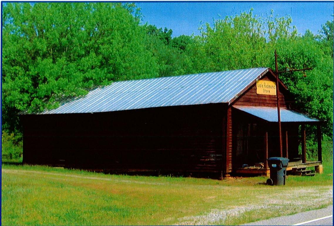
Figure 4. General store. Looking north from NC 115. East (main) and south elevations.
