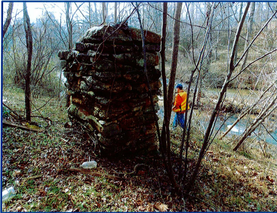
Figure 9. Redmond's Mill. One of three, free-standing stone piers that may have supported the flume or other appendage of the mill building (above). Road trace leading to mill site, looking north – general store visible in distant right background (below).
